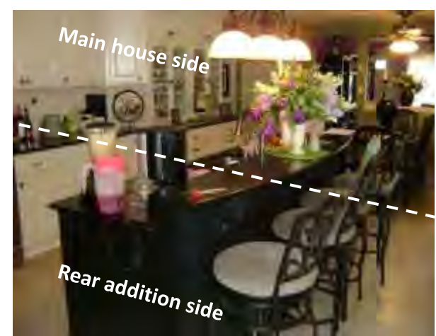
White dotted line represents location of original rear exterior wall of main house that separated rear addition.
