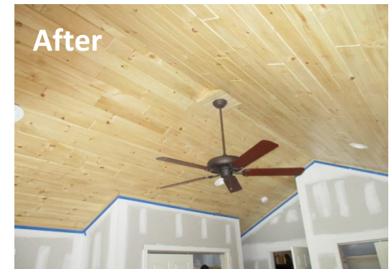
Completion of interior drywall, trim and ceiling planking
