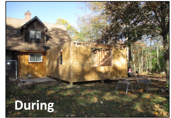
Erecting exterior walls
