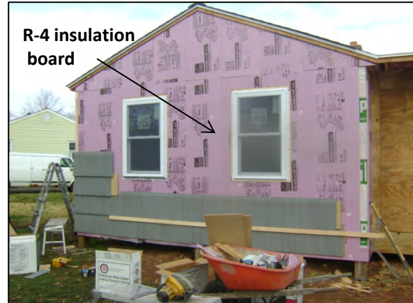
5) Shell & roof complete, windows installed and installation of exterior wood siding in progress.
