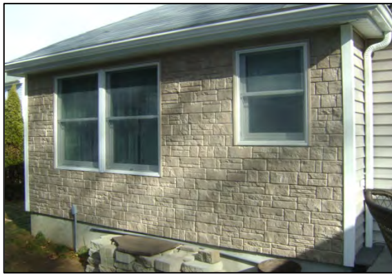
5) Completed , view of rear elevation. view , stone imitation vinyl siding.
