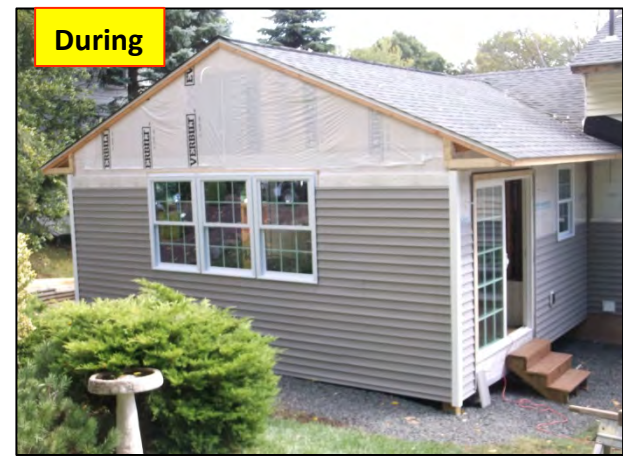
Roof shingled , windows / doors , start siding
