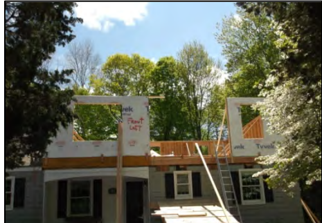
2:00 PM, Walls up, carry trusses.
