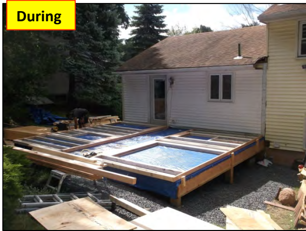
Footings excavated & poured , floor framed
