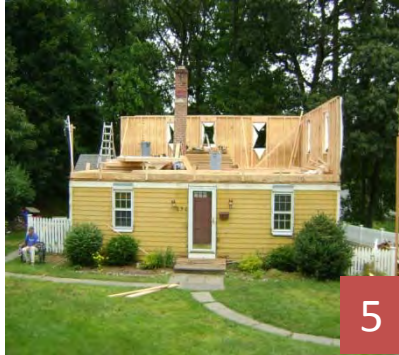
5. Continue erecting exterior walls ,50 % done by 1:30 pm.
