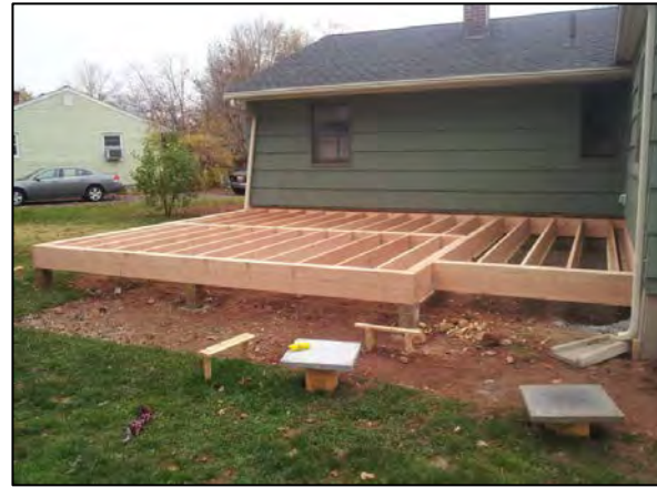
2) Entire floor structure build with 2 " x 12" ' boards for maximum depth for insulation.
