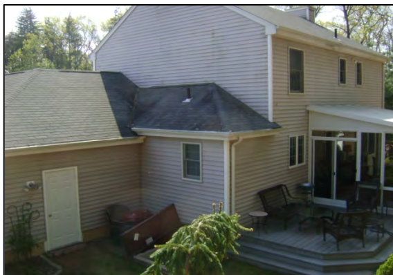
2) Before picture , rear elevation .
