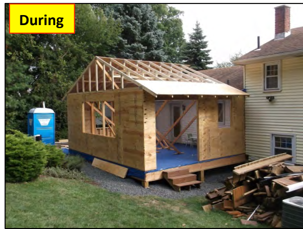
Walls & trusses erected
